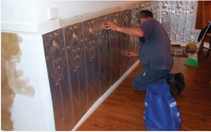
Marking out prior to installing
