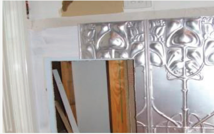
Panel cut out for A/C vent
