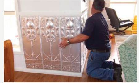
Panel folded returning around wall
